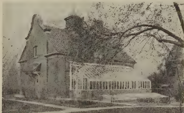
A brick garage with a two-compartment lean-to greenhouse and row of frames. The heating system in the garage can furnish heat for both structures. This type has no workroom. There is no door connecting the garage and the lean-to
